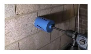
In all options; holes are drilled in the electrical room wall, and garbage area floor, to allow for the passage of wiring or conduits.
