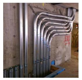
Large conduit would connect the MDP to the distribution panels via holes cut in the concrete wall and floor to lower parkade (Only 1 large conduit is required for our project)
